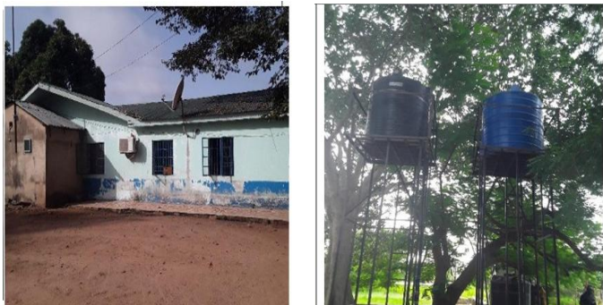
Facility to be renovated (Left) Proposed intervention sites (Right)
